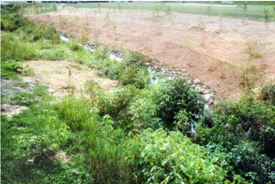
Figure 4. A graded stream bank allows for the establishment of riparian vegetation that will provide stabilization and habitat within the stream corridor.
