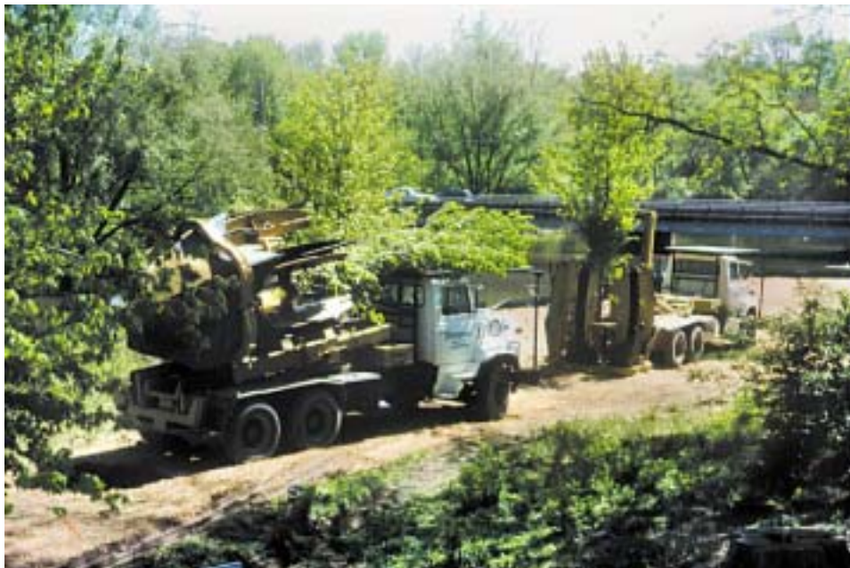
Figure 14. Seven 5" caliper red maple trees were planted to establish a transitional zone between the project site and the Gertrude Fox Conservation Area. This would allow for the "blending" of the project into the natural landscape.
