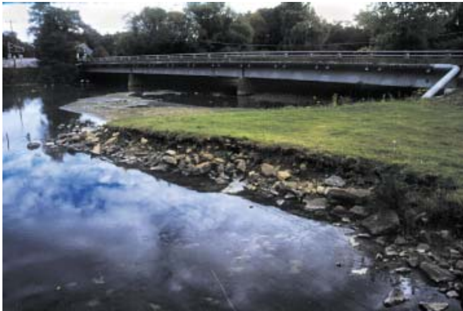
Figure 5. Mowing and waterfowl grazing of riparian vegetation has accelerated stream bank erosion adjacent to the spring raceway.
