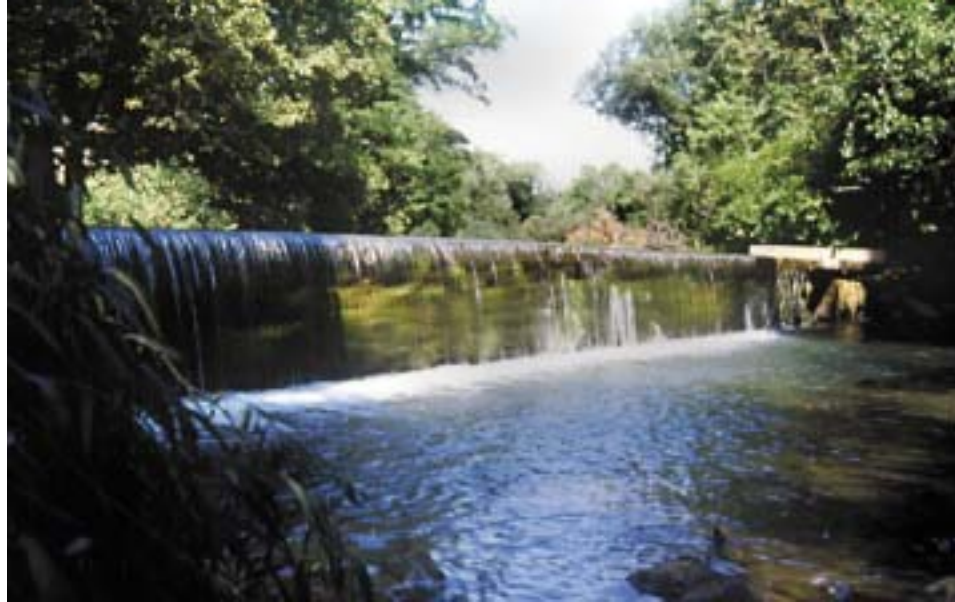
Figure 1. The low-head dam that is located immediately downstream of the project site has impacted the water quality and aquatic habitat of the Monocacy Creek.
