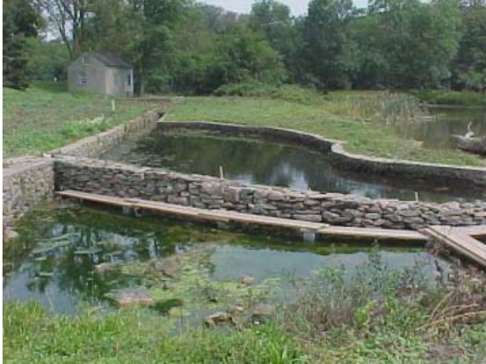
Figure 4. The spring raceway improvements were designed to provide stream bank stabilization and an enhanced cold water flow into the Monocacy Creek. A hand furnished stone wall was constructed to maintain the historical appearance of the property, while accomplishing these objectives.
