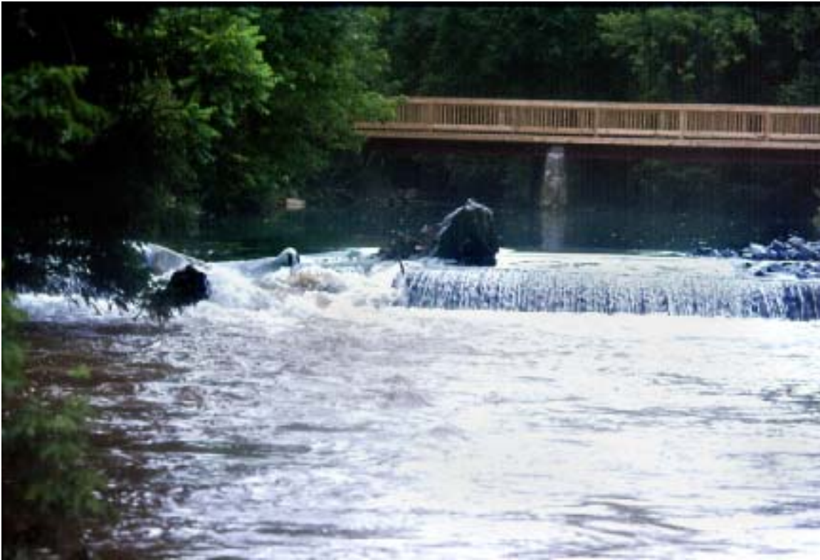
Figure 11. Breaching the dam caused a slow increase in the downstream water level by approximately three to four inches. The duration of this temporary rise in water level was approximately fifteen minutes and appeared to cause no negative downstream impact.
