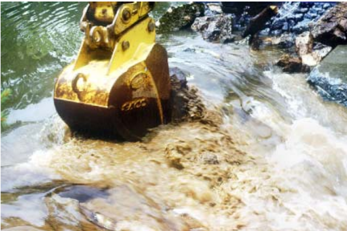
Figure 10. Removing the dam created a slight disturbance of the stream substrate within the project area. The long-term environmental benefits achieved by removing the dam should, however, negate this temporary disturbance.
