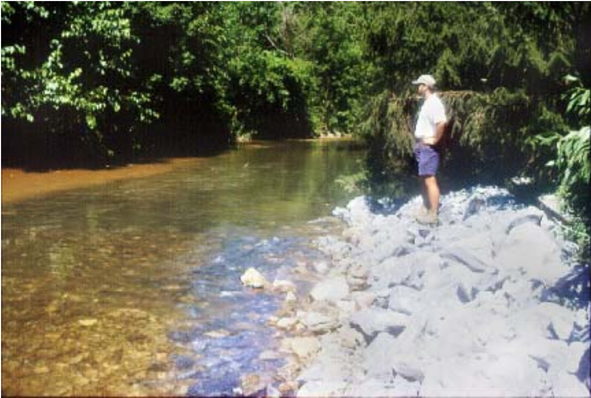
Figure 13. The stone that was used to stabilize the stream banks should vegetate and become camouflaged as sediment carried by the stream is deposited during storm events.
