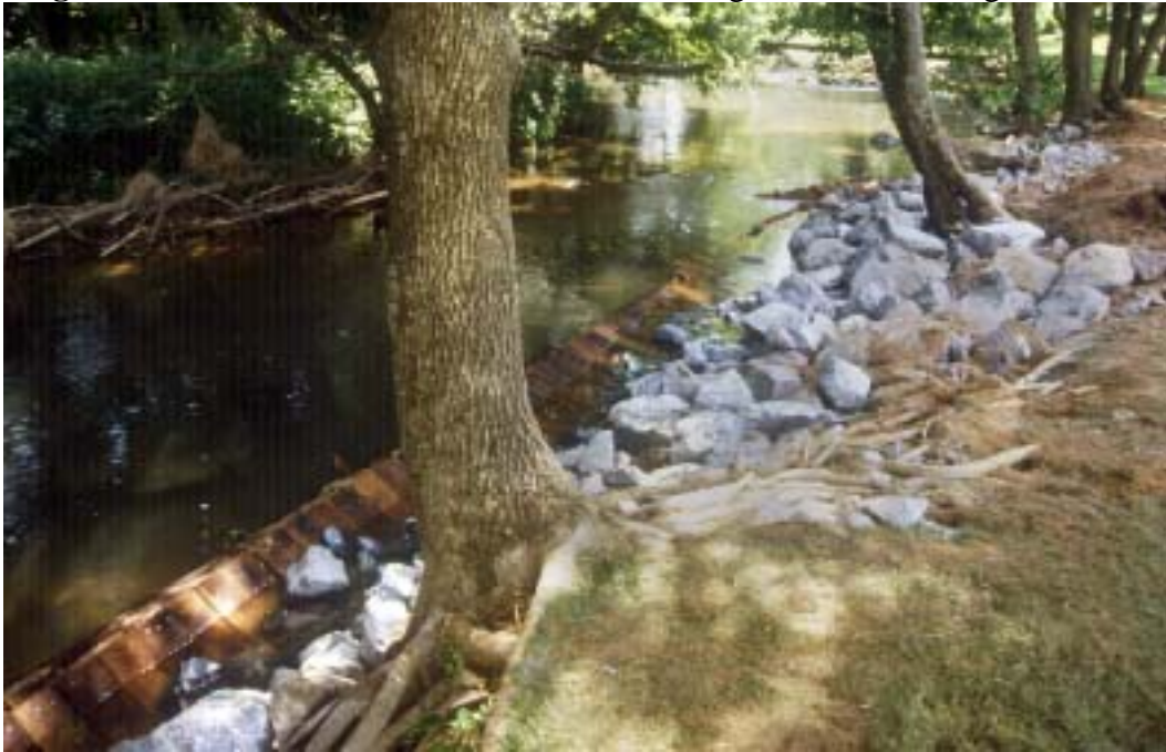
Figure 3 – Construction of modified bank cribbing with oak flooring and stone.
