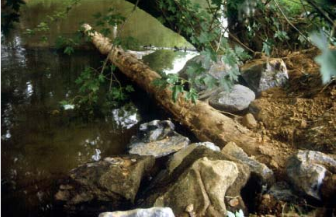
Figure 8 – Placement of a multi-log deflector directs water away from a severely eroded stream bank and imitates the woody habitat that was previously lacking in this section of the Little Lehigh Creek.
