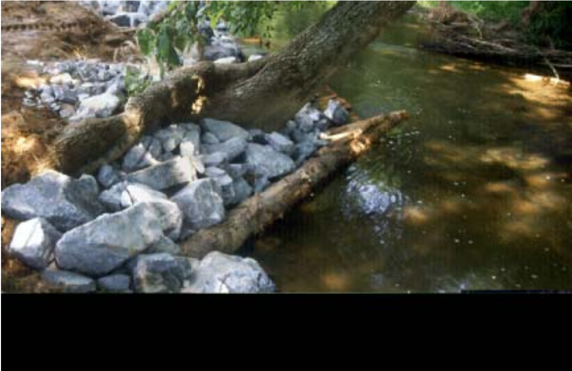
Figure 1 – A stacked deflector with oak flooring provides overhead cover for fish and narrows the stream channel.
