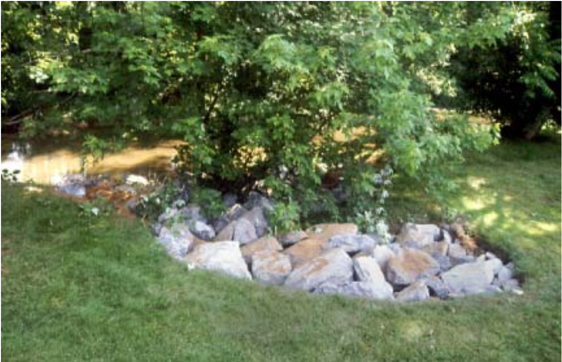
Figure 9 – Stone was used to stabilize this eroded area adjacent to the multi-log deflector. The area was contributing silt to the stream and was negatively impacting aquatic habitat.
