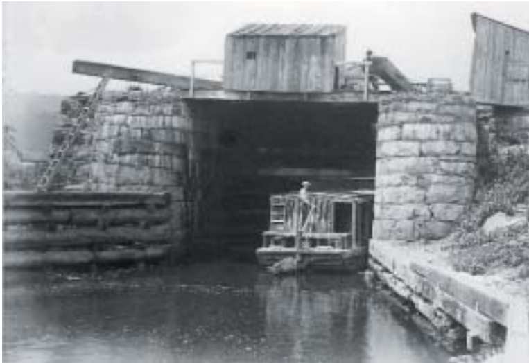
Some locks in the 26-mile Upper Grand Section of the Lehigh Navigation were as high as 40 feet. In this section there were only eight short canals. Mostly it consisted of high-lift locks and dams. The boats traveled between the dams in the slack-water pools created by the dams. From the collection of the National Canal Museum, Easton, PA.
