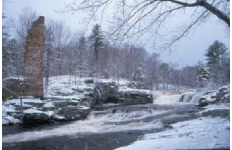
Protected recently by a local visionary, Commander John Butler, this historic grist mill at Stoddartsville, Luzerne County (near Blakeslee) was built to take advantage of the new Lehigh Navigation. Unfortunately, the northern terminus of the system was established 12 miles downstream in White Haven.
