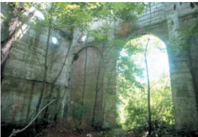
The remnants of the Thomas Iron Works in Hokendauqua, Lehigh County, are adjacent to the Lehigh River. This was the first plant in the country to burn anthracite coal successfully.
