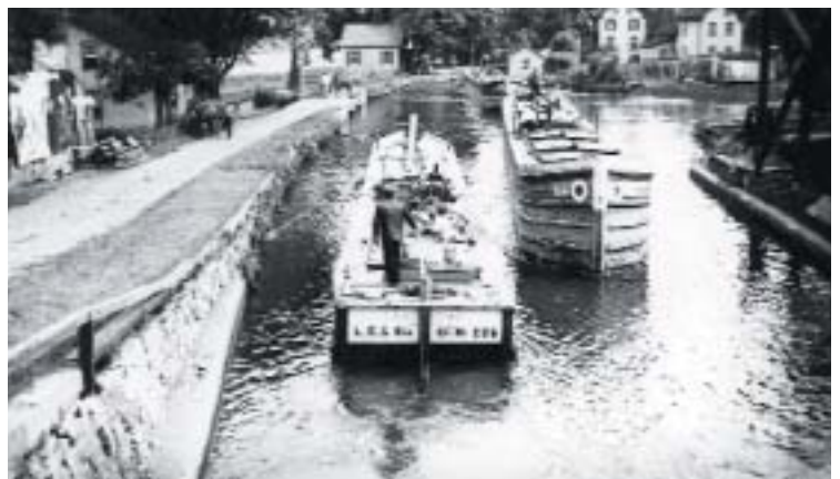
Six feet deep, 60 feet wide at the top, and 45 feet wide at the bottom, the canals of the Lehigh Navigation were built to allow two boats to pass each other. From the collection of the National Canal Museum, Easton, PA.
