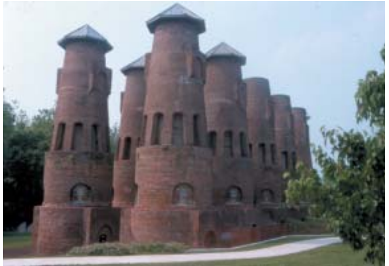
A high-quality limestone was discovered in the Lehigh Valley during the construction of the Lehigh Navigation, and the American cement industry was spawned. These kilns, located in Saylor Park, Lehigh County, were used in the process of making limestone into Portland cement.
